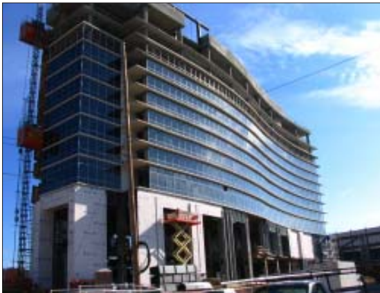
New Hilton Hotel under construction in Downtown Branson
